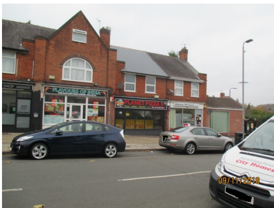
113 to 117 Central Avenue
