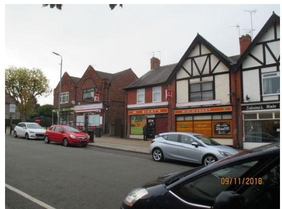
97 to 103 Central Avenue
